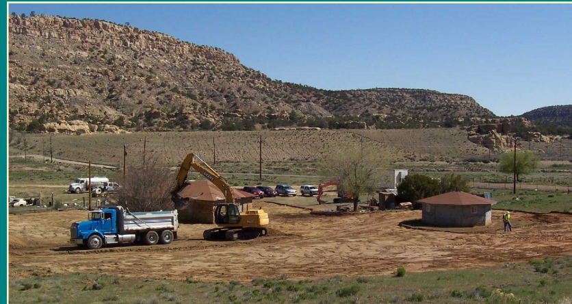
Radium-contaminated soil removal, Red Water Pond Road, 2007; partially reclaimed abandoned mine in rear
